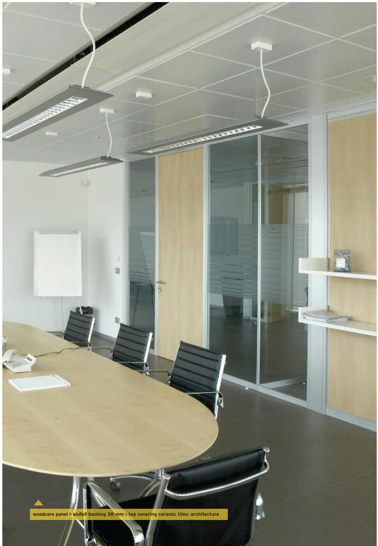
woodcore panel > alufoil backing 38 mm > top covering ceramic tiles: architecture
